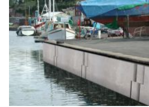
Water proofing piers
