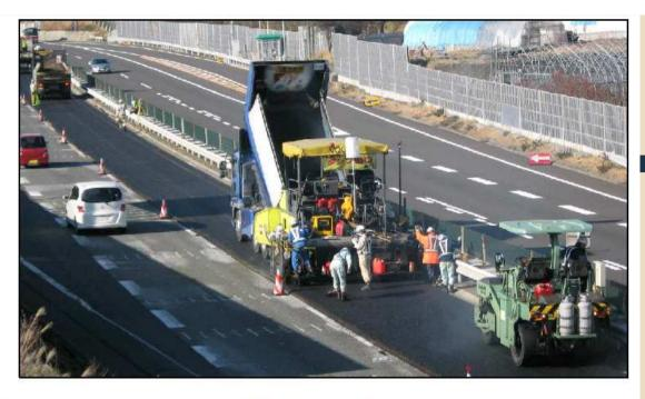
Photo 6: Paving work of 3D-MC asphalt paver at expressway overlay
