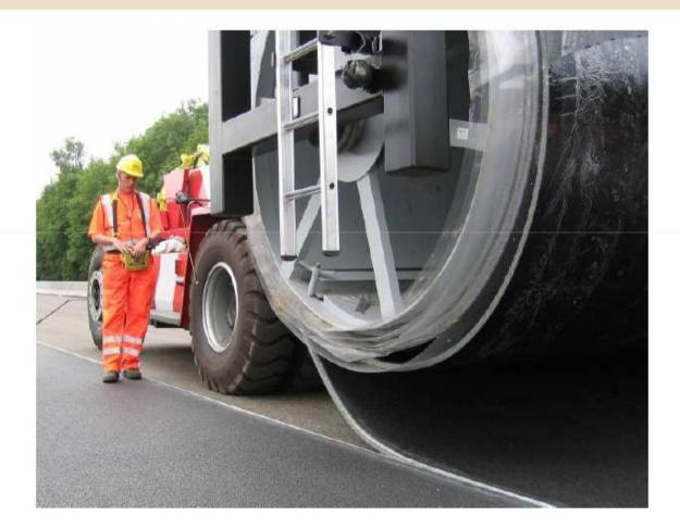
Figure 5: The operator controls the movement of the asphaltmat and places it very precisely.
