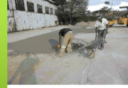
Figure 3Placement of RCC material
