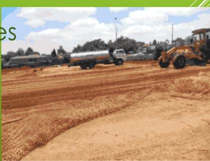
Figure 4Preparation of sub grade
