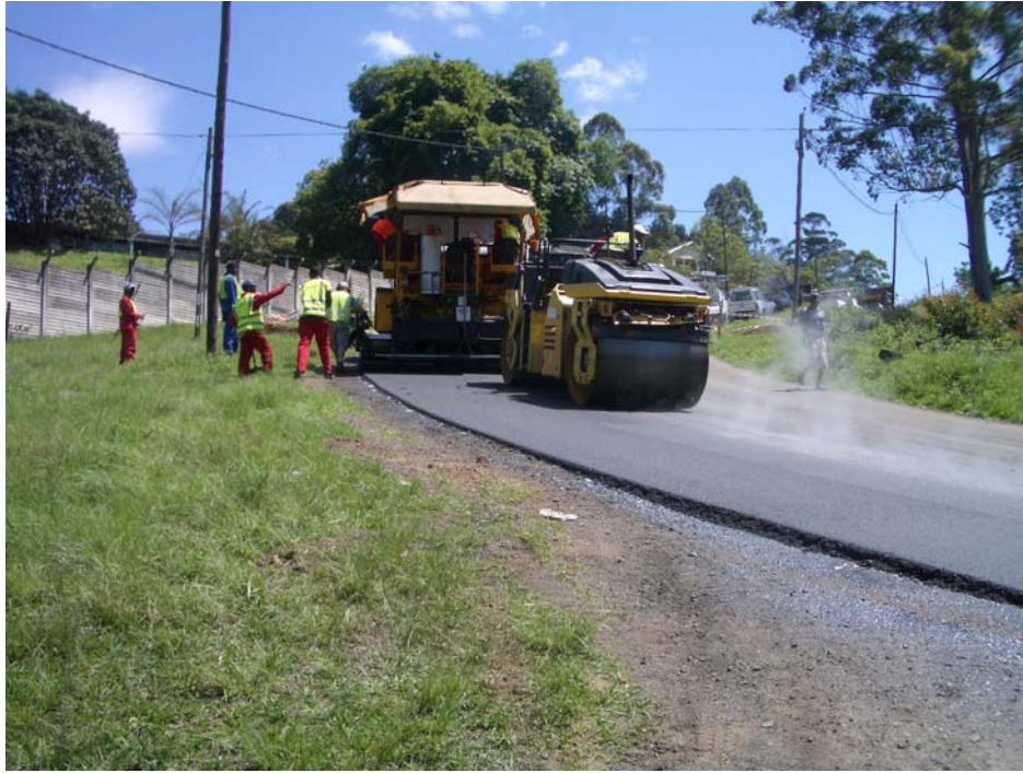
Paving up steep grade using mix containing 30% RA
