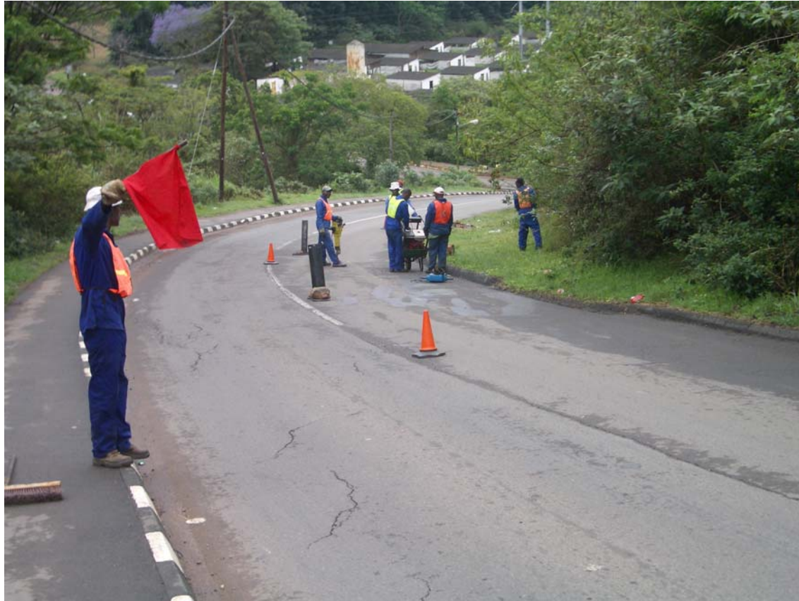
Patching the severely distressed areas
