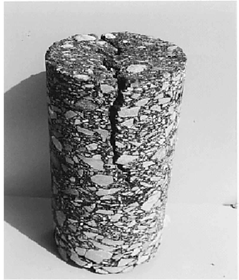
Photograph 2. A Core of Top-down Crack
