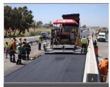
SURFACE DEEP Bitumen emulsions' ability to be applied cold and without the use of hydrocarbon fuel for heating drastically reduces the release levels of harmful gasses into the atmosphere.
