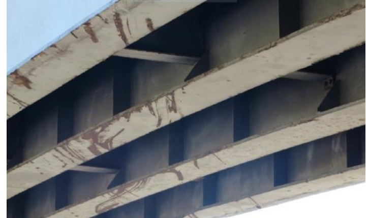
Evidence of impacts on bridge deck
