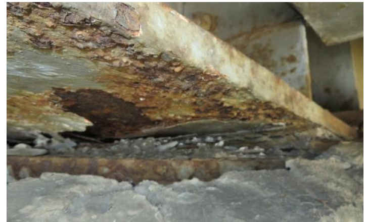
Evidence of impacts on bridge deck
