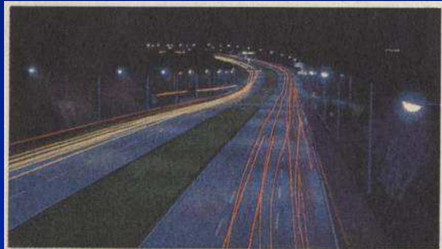
Concrete cuts highway lighting costs. Studies show proper lighting levels can be reached on concrete with 50% fewer fixtures than needed for dark-colored pavement.
