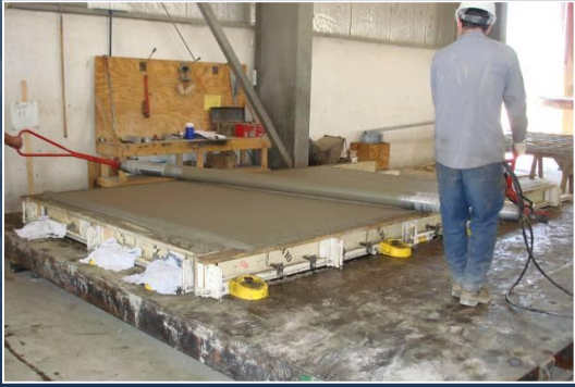
Roller Screed Insures Accurate Top Surface
