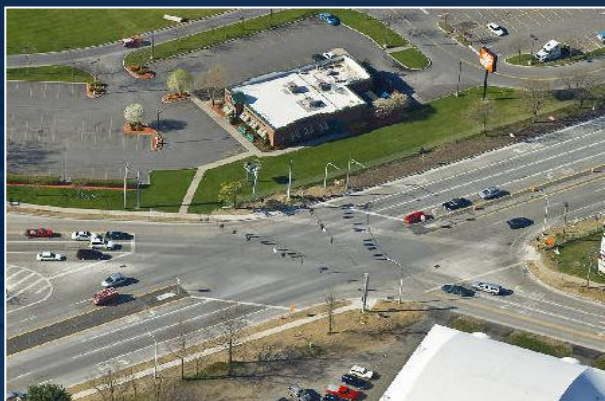
Replaced in 17 Nights!
