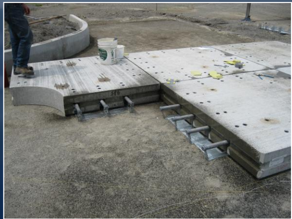
Independent Dowels Placed in Slots
