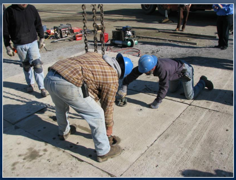
Be Sure Surfaces Match Before Unhooking
