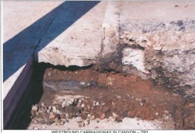
WESTBOUND CARRIAGEWAY IN CANYON – TP1
