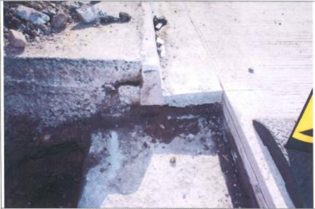
WESTBOUND CARRIAGEWAY IN CANYON – TP1
