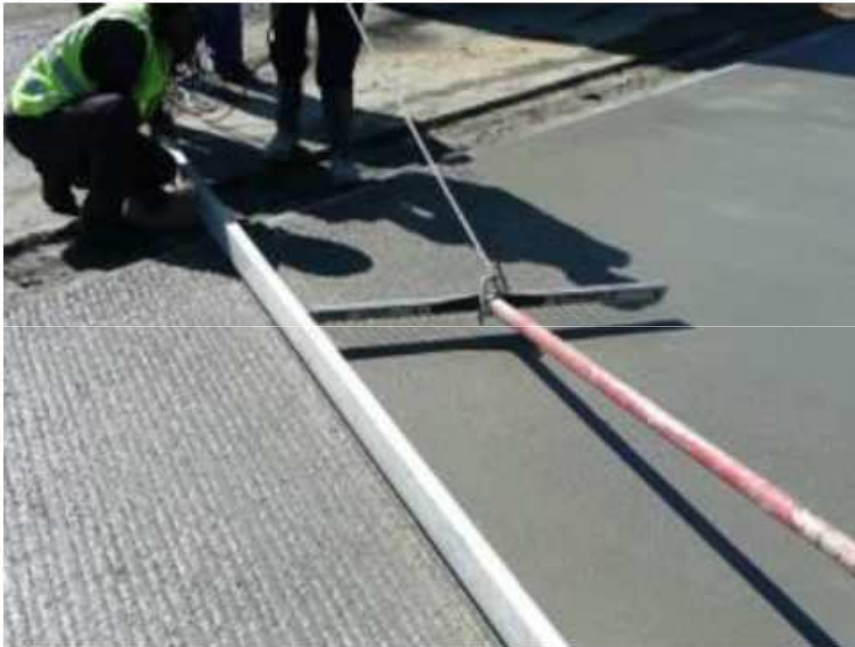
Figure 10 – Application of textured finish – note good texture after hardening.
