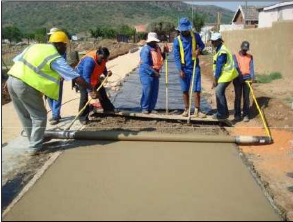
Photo 14 - Roller screed in use at Mamelodi
