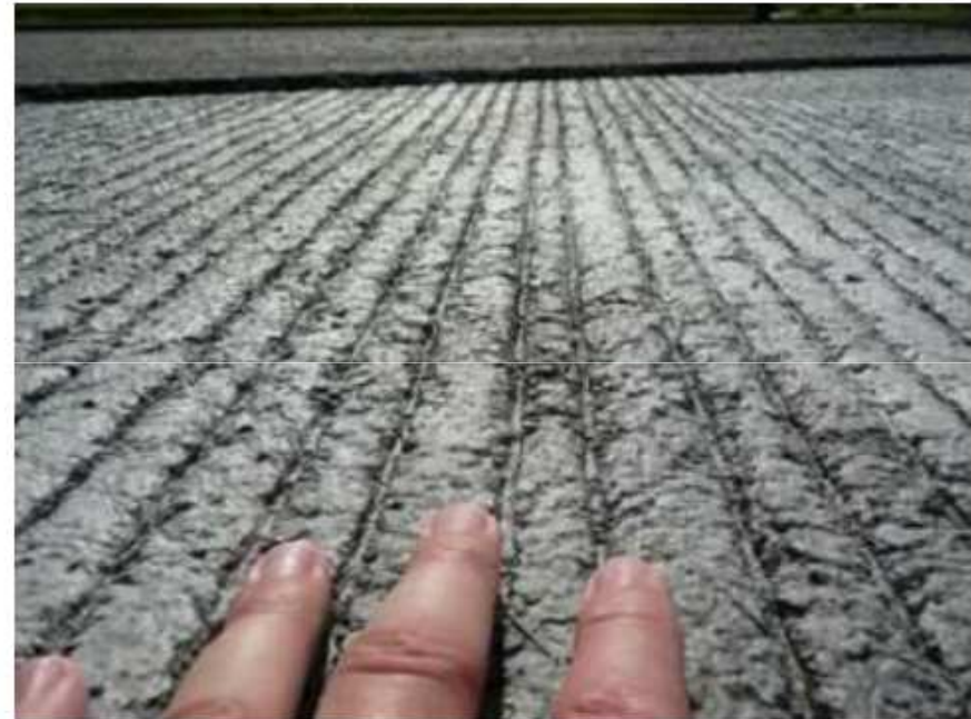
Figure 10 – Application of textured finish – note good texture after hardening.
