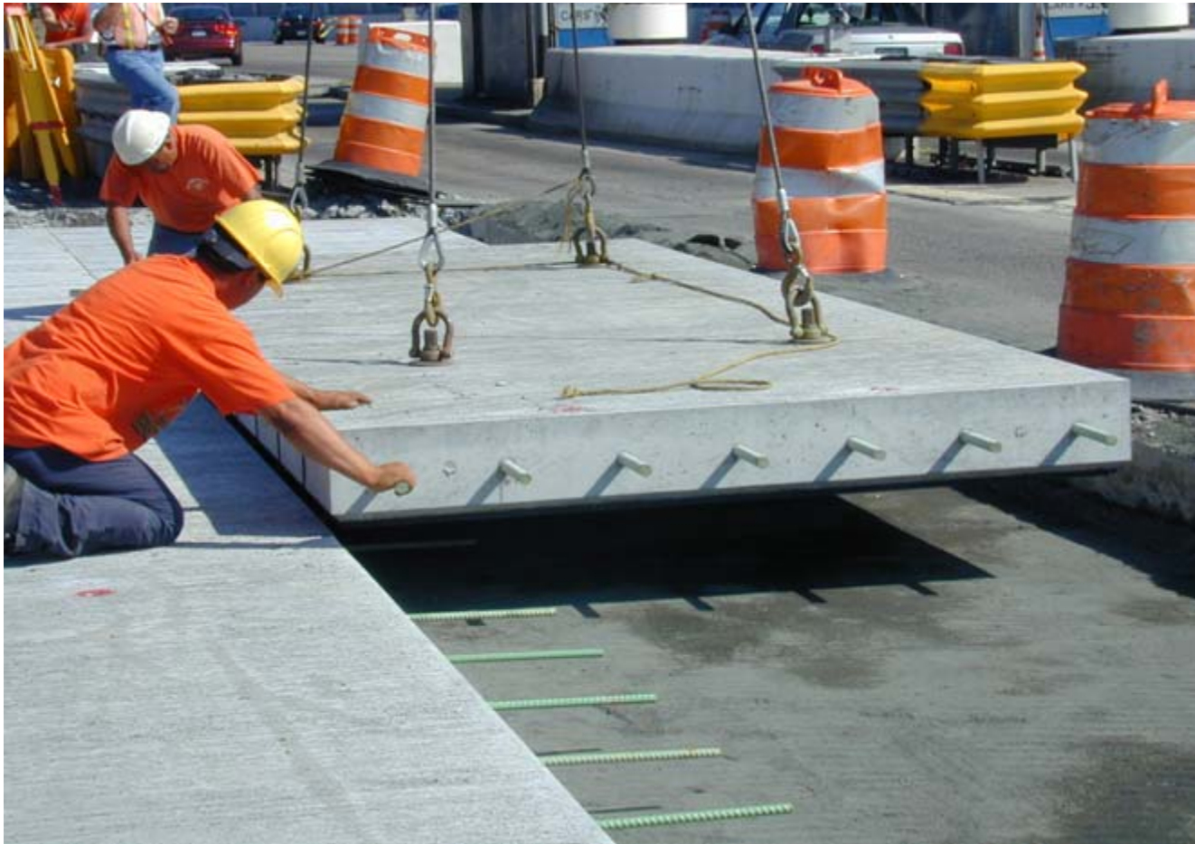
Pre-cast concrete slab replacement
