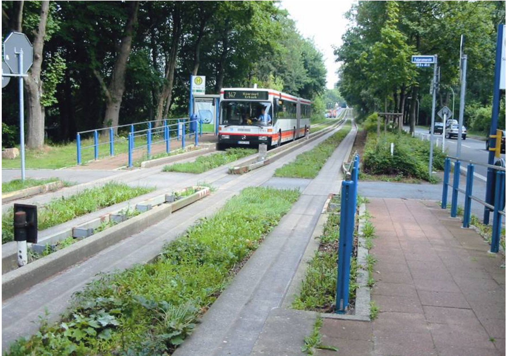
Guideway crossing, Essen, Germany
