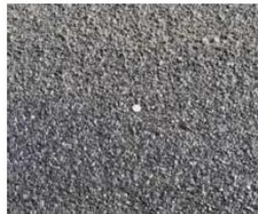
b) 3/8 inch Chip Seal Mat, Post Construction, Sept 2010
