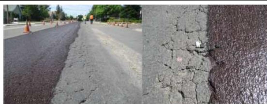
Figure 7. Placement of the microsurfacing leveling course over wide cracks, Turlock, CA, 2010
