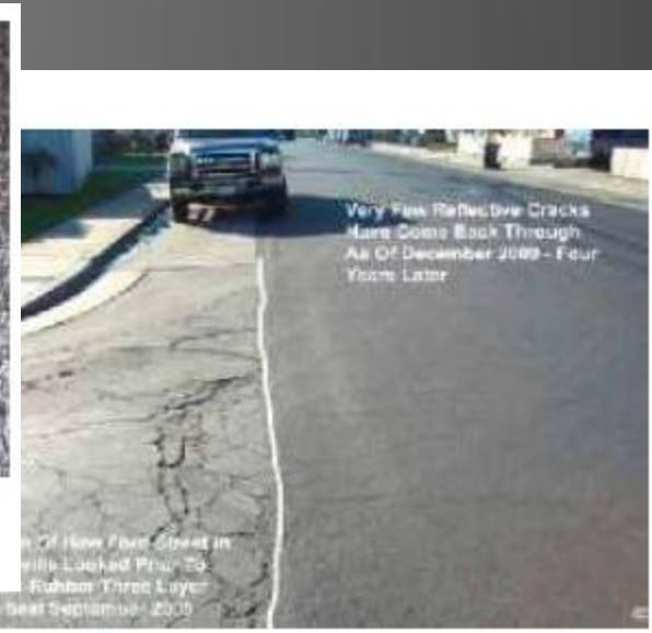
Figure 16. Asphalt rubber 3-layer system, Ford Street, Watsonville, CA, 2009 (4 1/2 years later resisting cracking)
