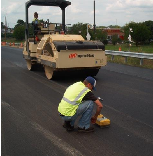
Compaction & density achieved by the contractor on site
