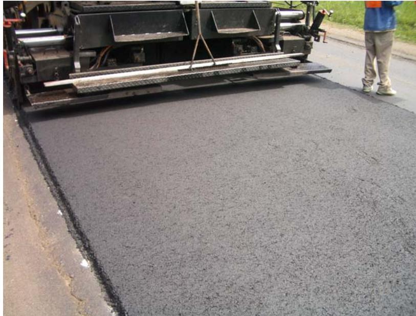
“Recycled hot-mixed asphalt containing RA has the same quality and performance requirements as mixes using all new materials”
