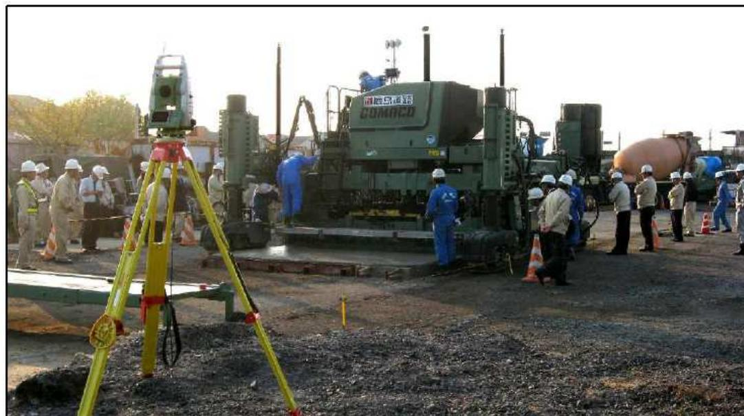
Photo 7: Trial work of 3D-MC slip form paver for concrete paving
