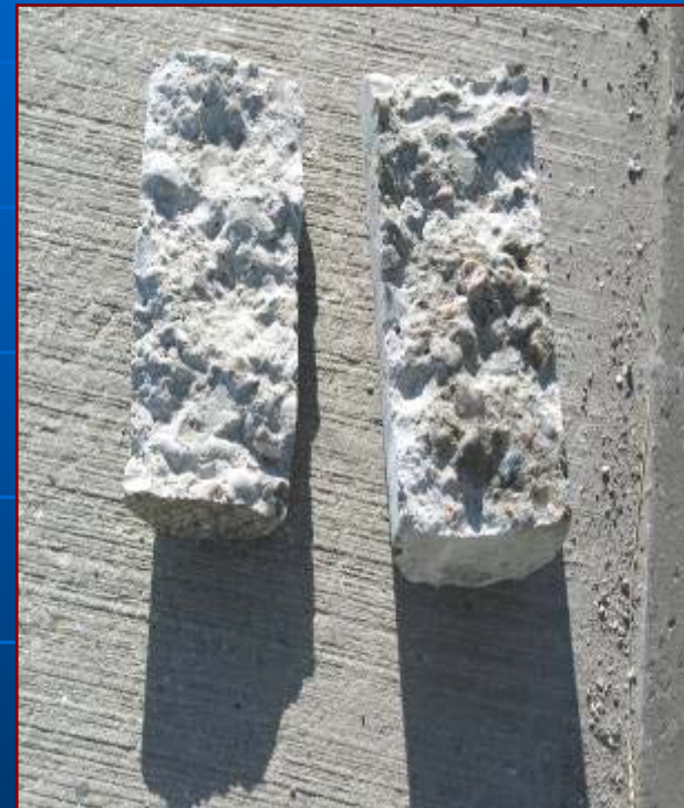
Broken core showing good aggregate interlocking Crack should be vertical throughout depth of core
