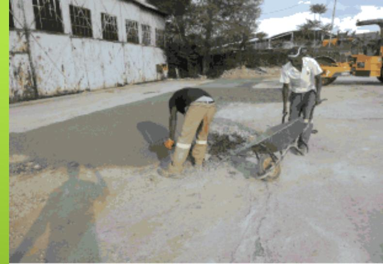
*Figure 3 Placement of RCC material*
