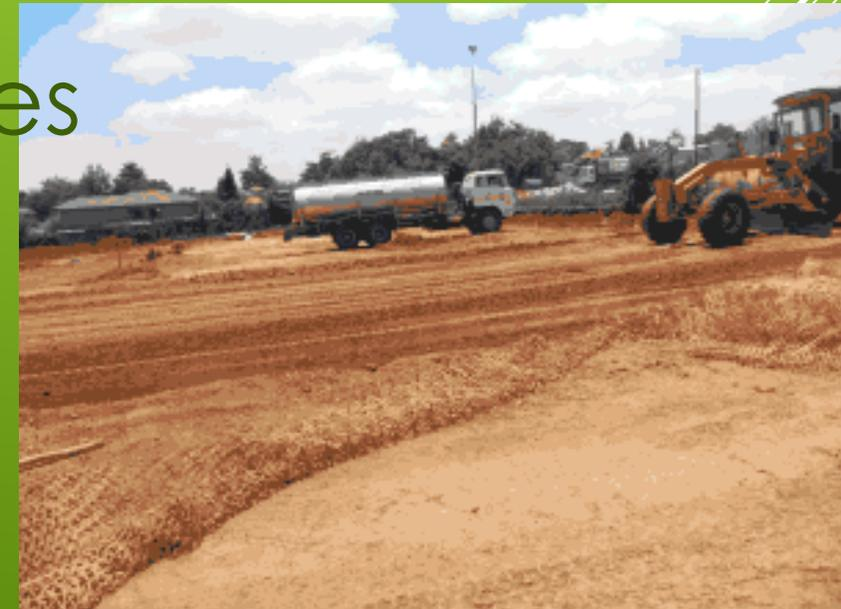
*Figure 4 Preparation of sub grade*
