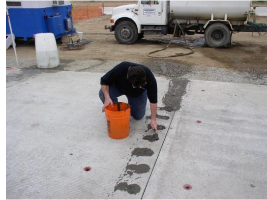
Excess bedding grout pouring from the exit hole
