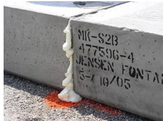
Expanding foam used for sealing of the outer edges of the joints
