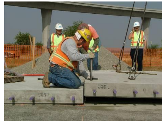
Placement of the slab on the adjacent lane
