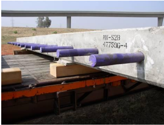
Female end of the tie-bars cast into the longitudinal edge of the slab
