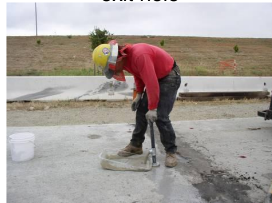
Excess bedding grout pouring from the exit hole
