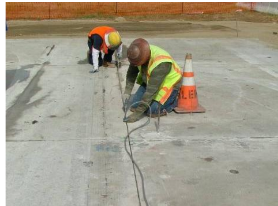
High density foam strip installed in the joints
