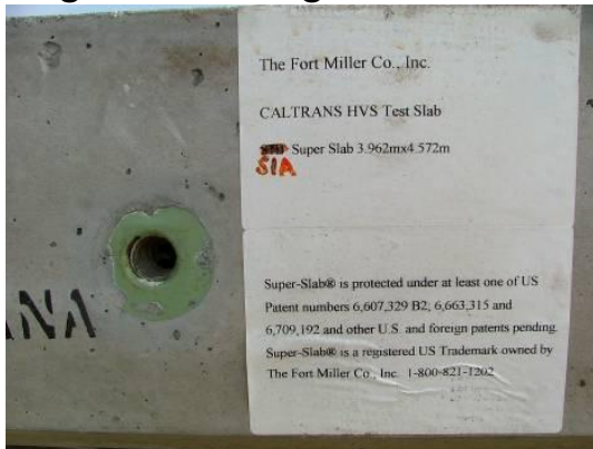
Female end of the tie-bars cast into the longitudinal edge of the slab
