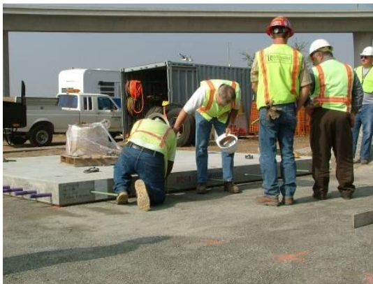
Fixing the tie-bars on the longitudinal edge
