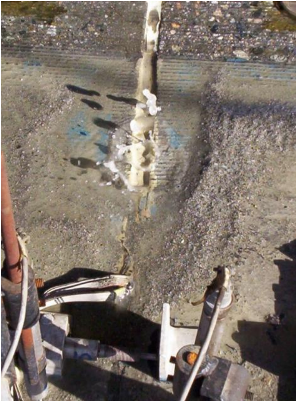
Pumping through the joint
