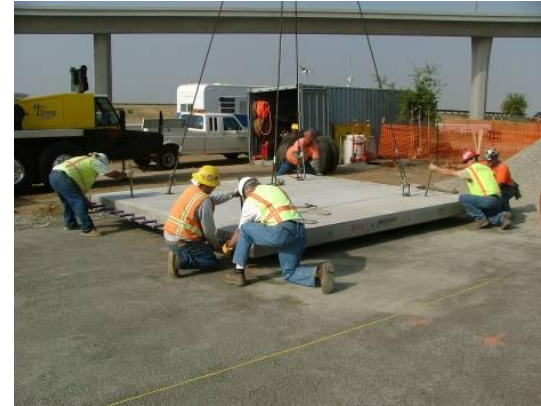
Placement of the slab on the adjacent lane
