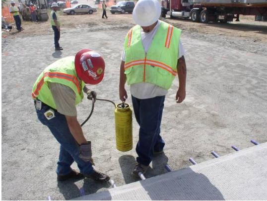
Spraying of the dowel-bars with a bond-breaker
