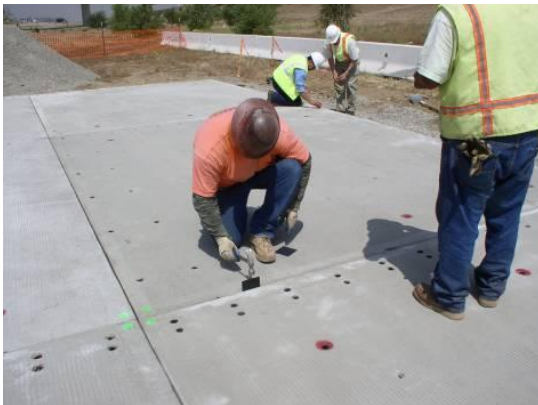
Plastic spacers being driven into the joints between the un-grouted slabs
