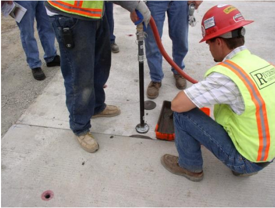
Filling of the dowel and tie-bar cavities with grout
