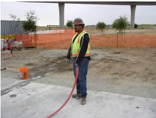
Injection of the bedding grout
