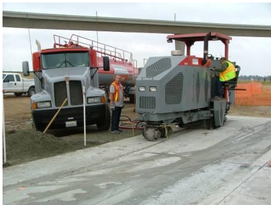
Level grinding of the surface
