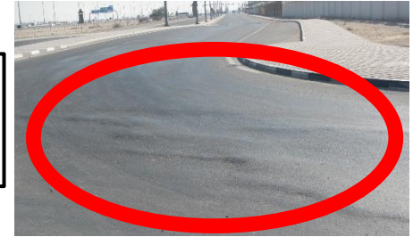
Pavement Deformation
