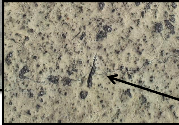
Corner curling of debonded slab after construction
