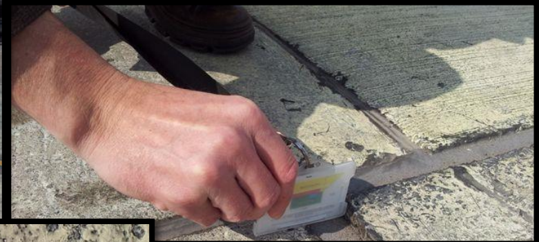
Corner curling of debonded slab after construction
